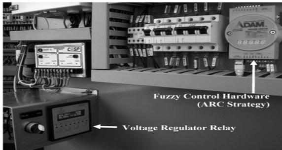
Figure 12 real fuzzy controller in substation
